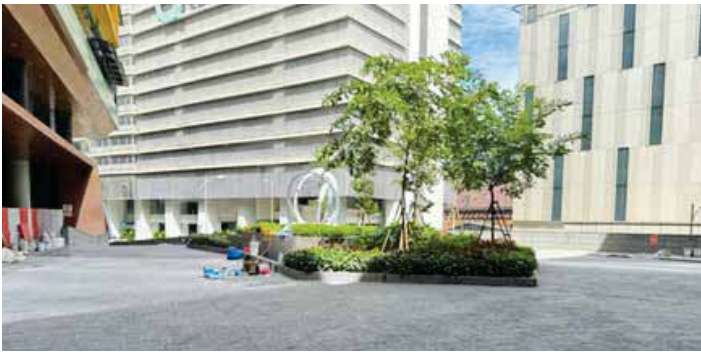
Figure 16: Platinum Sentral - After upgrading works
