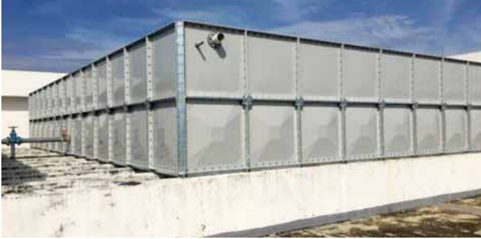
Figure 15: Sentral Building 4 – Finished installation works of new FRP Water Tank for HSE initiative
