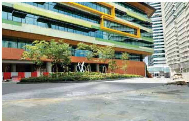
Figure 19: Platinum Sentral - Main entrance lobby drop off - upgrading works in progress
