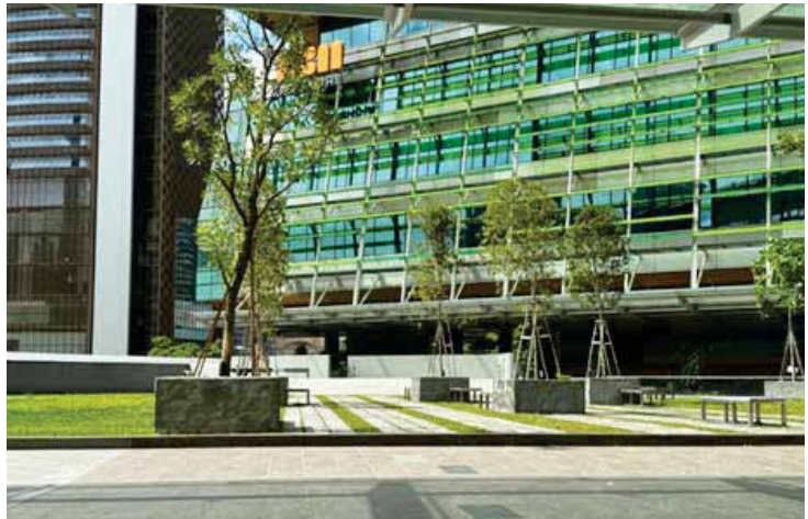
Figure 17: Platinum Sentral - West Courtyard after upgrading works
